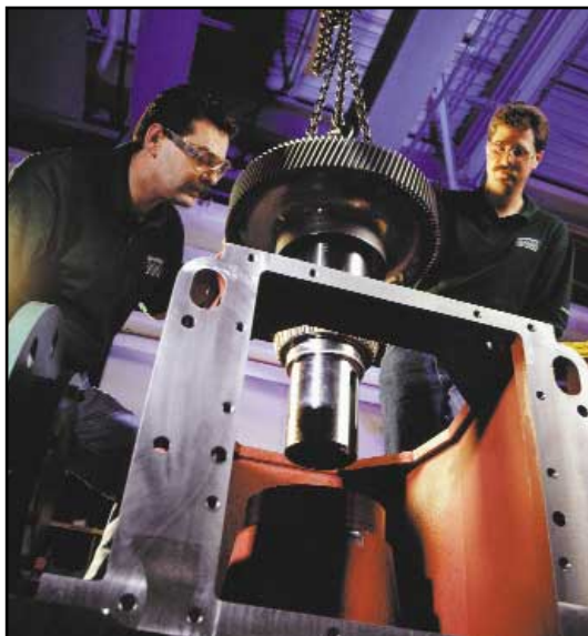
Reassembly of a 700 series reducer after repair.
